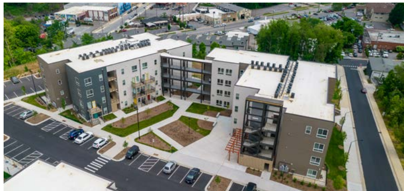
Photos this page / next: The Lee Walker Heights Development (now named Maple Crest). Images courtesy of Mountain Housing Opportunities and McMillan Pazdan Smith Architecture.
